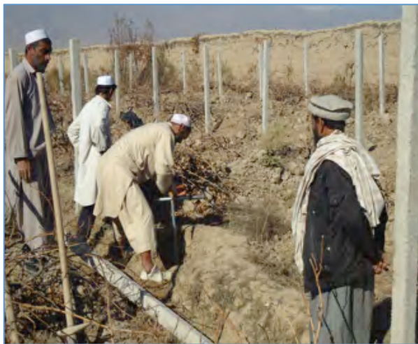
Training farmers on post installation with ground auger, Kabul
