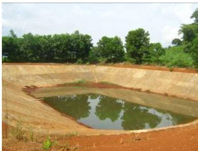
Picture 3 Bed and surroundings of the reservoirs were concreted but water is not enough for running the dripping system
