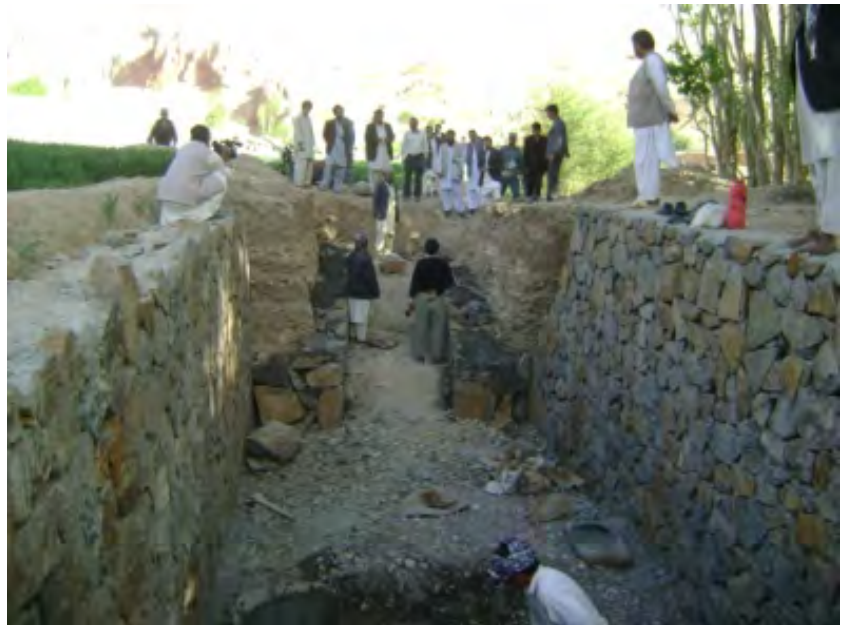
Partially constructed potato cellar in Bamyan, 2011.
