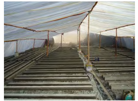
Posts curing under plastic due to cold weather
