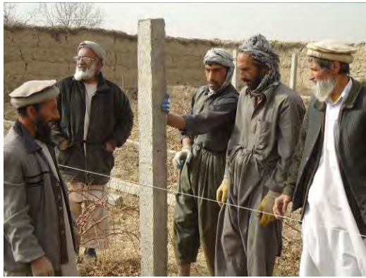
Installing posts in Shamali
