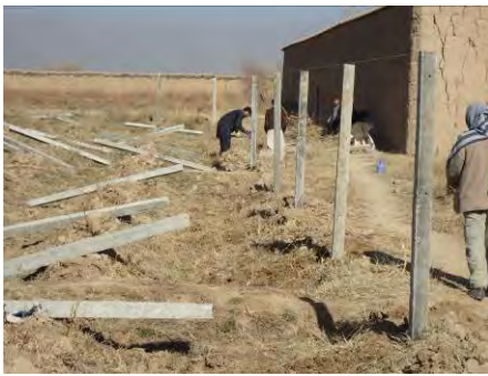
Installing posts in Shamali
